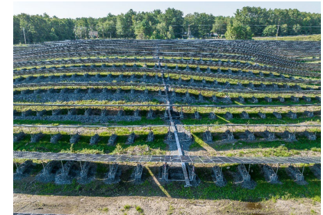
6.1 MW, Geoballast Wells, ME
